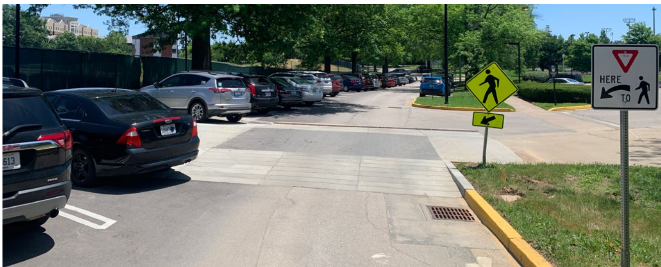
Figure 5.8 Complex Drive raised crosswalk and angle parking
